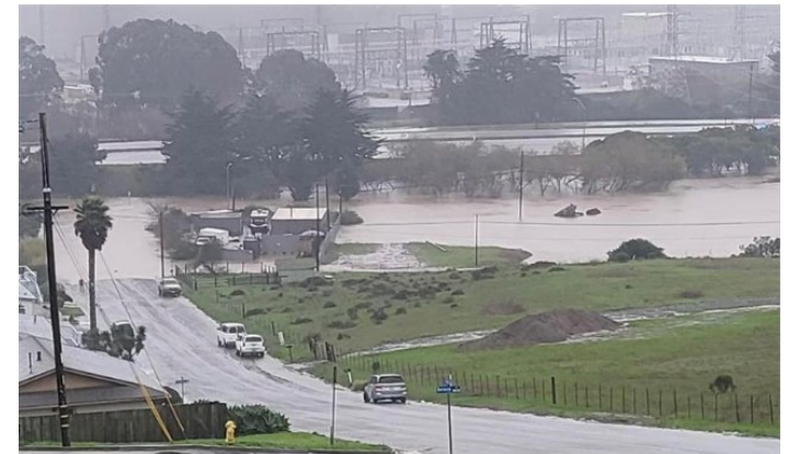
Flooded substation in Morro Bay, CA, January 2023.
